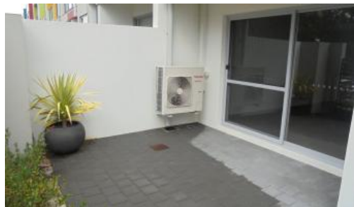
21, 30 Lambeth Circle, Wellard
