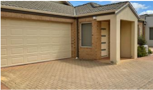
Unit, 3/17-21 Third Avenue, Kelmscott
